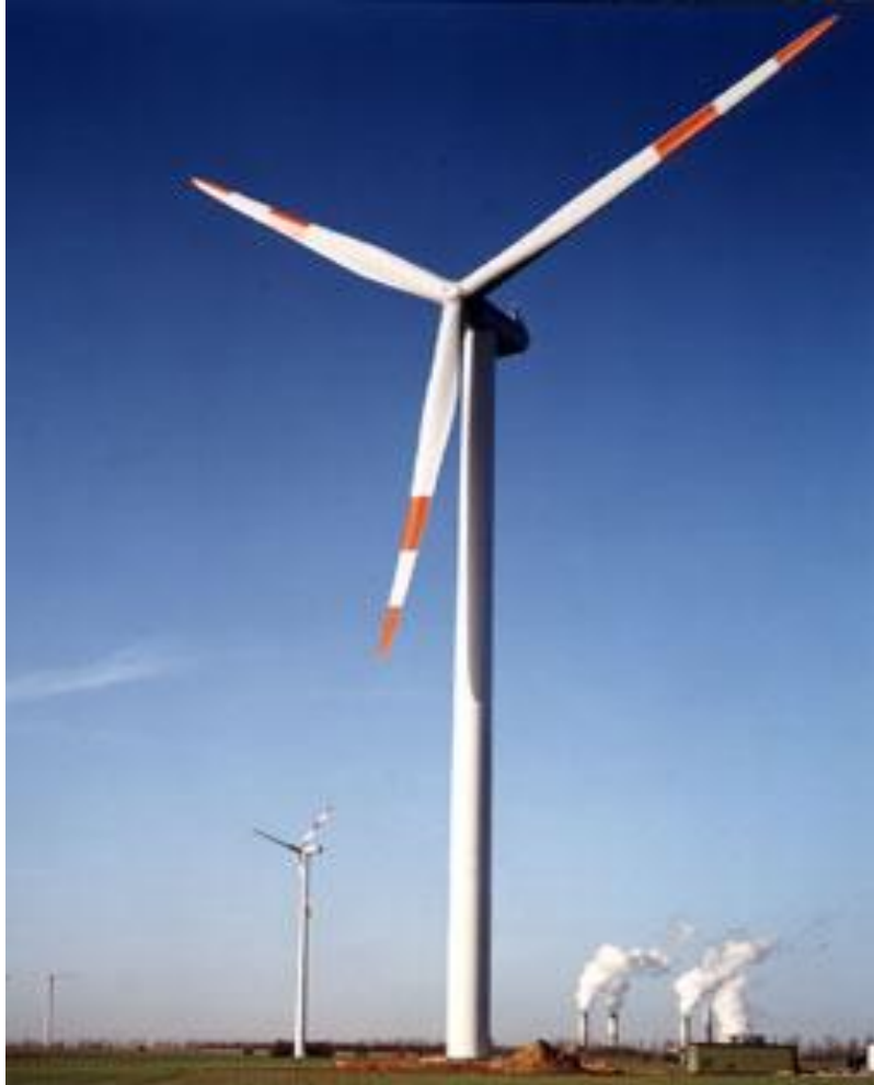
2.5 MW Nordex wind turbine (80-m tall) Grevenbroich, Germany
