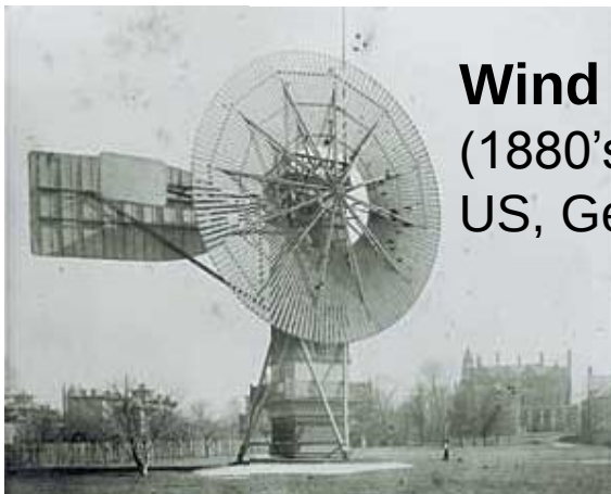
12kW DC Turbine Cleveland, USA 1887 (C.F. Brush)
