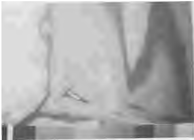
Figure 1-9B. Infrared Thermograph of Same Corner Reveals Interior Wall to be Several Degrees Colder. Dip in the Pattern is First Vertical Stud, Separating Two Pockets of Cold Air.
