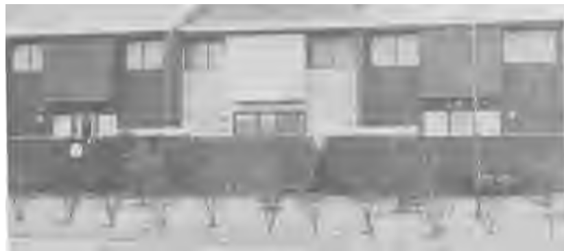
Figure 1-11B. Early Morning View of Frost Pattern on Back Slopes of Attics of the Three Highly Instrumented Townhouses at a Time when the Middle One has not yet Received Retrofit Package A. Dark Color Indicates Greater Heat Flow Through Roof and Less Frost Formation.
