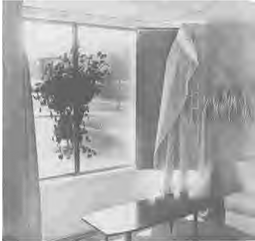
Figure 2-7A. Insulating Shutters in South-Facing Living Room Window. Curtain was Fastened Directly to Shutters.
