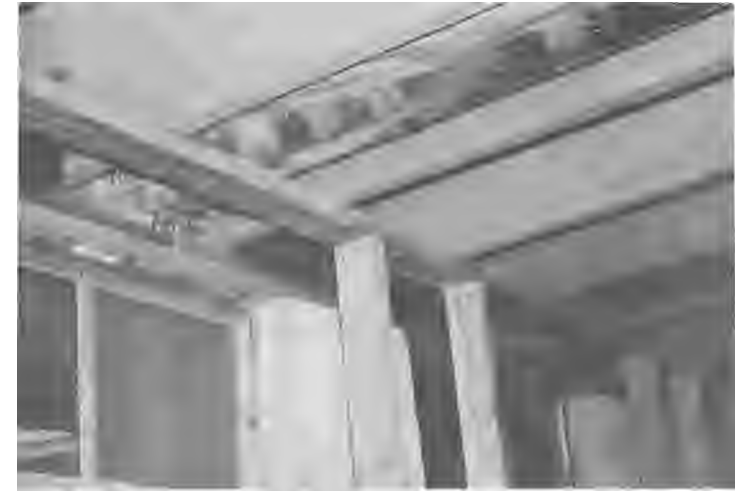
Figure 1-6C. Insulation of Duct and Overhang, Part of Princeton Retrofit Package C.
