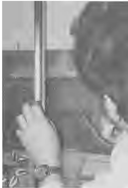
D: Kenneth Gadsby Installs Weatherstripping in Sliding Panel of Patio Door, Part of Princeton Retrofit Package B.
