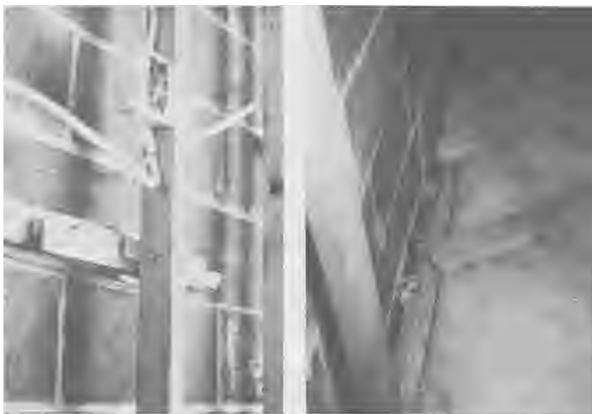
A: Seen at Time of Construction, Downstairs.
