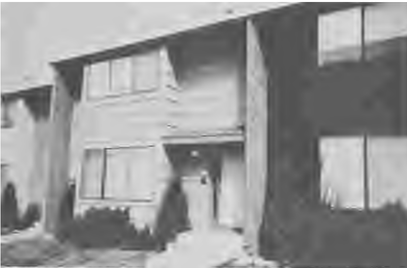
Figure 1-2B. Front View of Quad II Townhouse Rented by Princeton. Masonry Firewalls Project Beyond the Structure in Brick; Central Projection (with Windows of Living Room and Master Bedroom) Terminates One Foot Above Ground Level (Behind Bushes).
