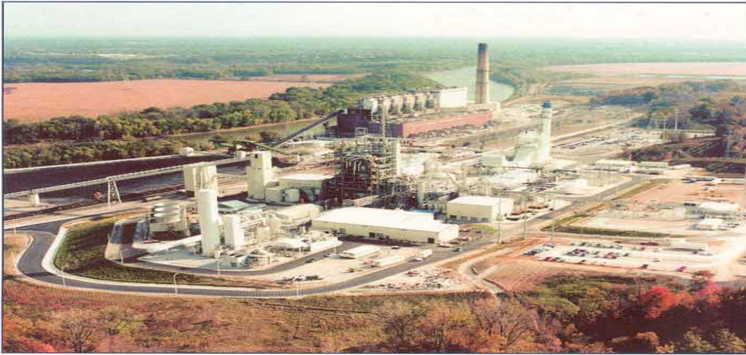
The Wabash River Coal Gasification Repowering Project
